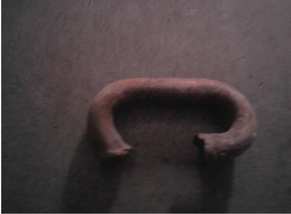
Figure 3. Bridle chains link broke at weld portion.
