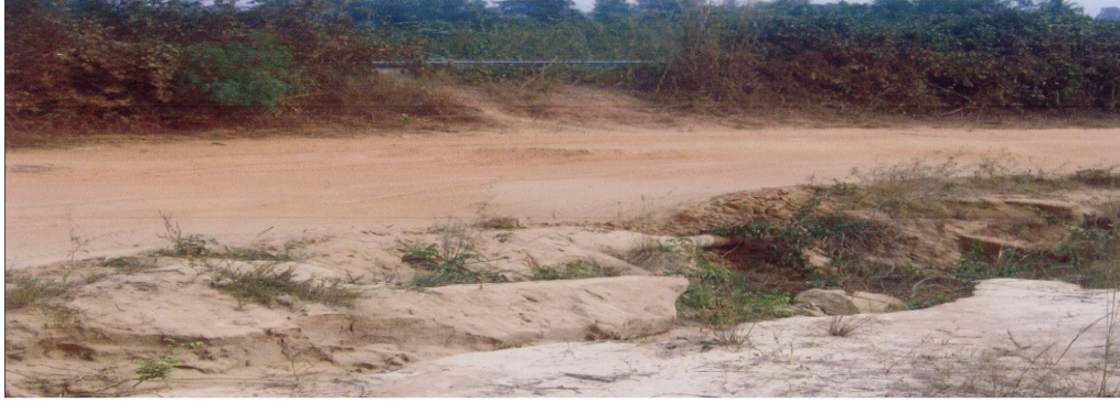
Figure 7. Effect of an exhausted quarry runoff that threatens the rails of Adétikopé.
