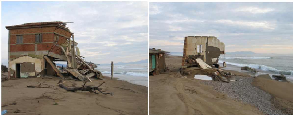
Figure 13. Intense erosion phenomena of the coastal zone - regression of the shoreline (Epitalion in the south-east of the Alfeios river estuaries) (Mertzanis, 2010).
