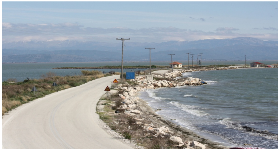
Figure 10. Thin sand barrier between Logarou lagoon and Amvrakikos Gulf; has distinguished the coastal protection works along the shoreline (rock armour, riprap, etc.) (Mertzanis, 2011).
