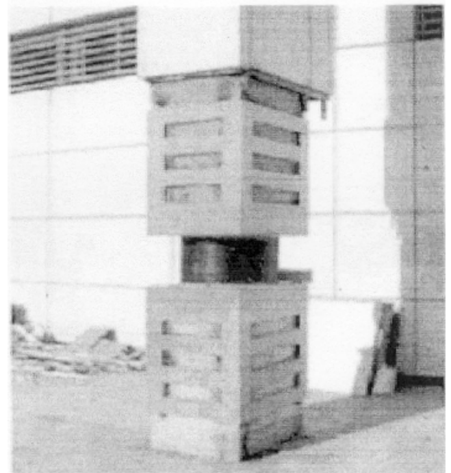
Figure 25. Steel jackets replacing severed reinforcing bars.
