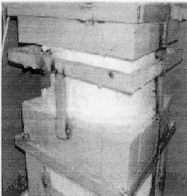
Figure 26. Installation of fire proofing elements.
