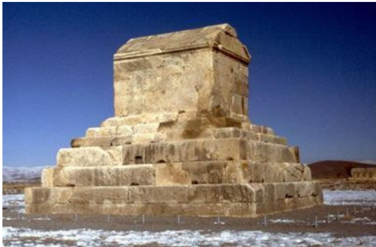
Figure 2. Mausoleum of Cyrus, the oldest base-isolated structure in the world.
