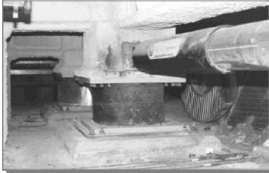
Figure 20. Isolator installation in building.
