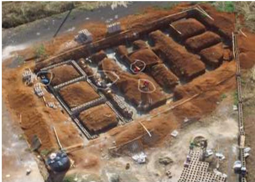
**Figure 5.** Worker in the foundation working without their personal protective equipment and the foundation basket dropped carelessly on the floor, captured by a DJI Phantom 3 Standard drone.
