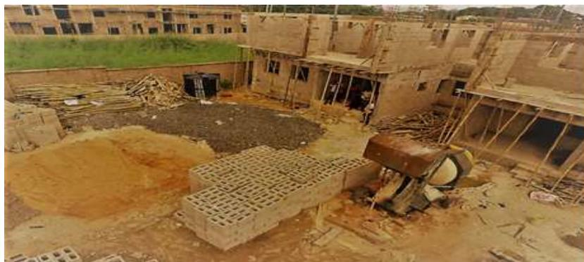
**Figure 8.** Aerial reality image of material and equipment onsite during closing hour including offcuts scattered on the floor. captured by a DJI Phantom 3 Standard drone.
