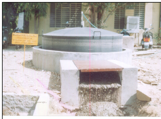
Figure 4. Jatropha based biogas plant (floating drum type).
