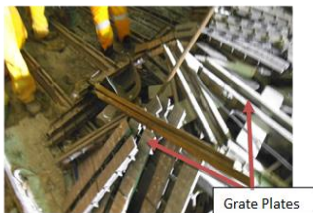
Figure 2. Cooler undergoing maintenance.
