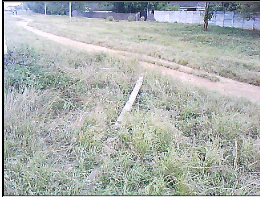
Plate 4. Fallen pylon: A common feature in Marlborough East.
