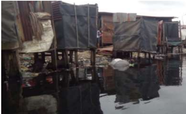
Plate 5. A typical toilet system in Makoko.
