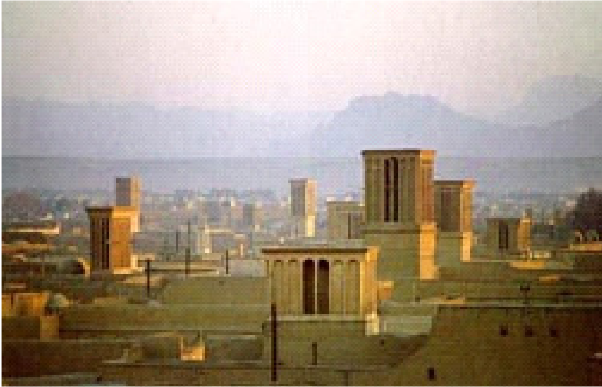
Figure 1. A view of the four sides' ventilator.
