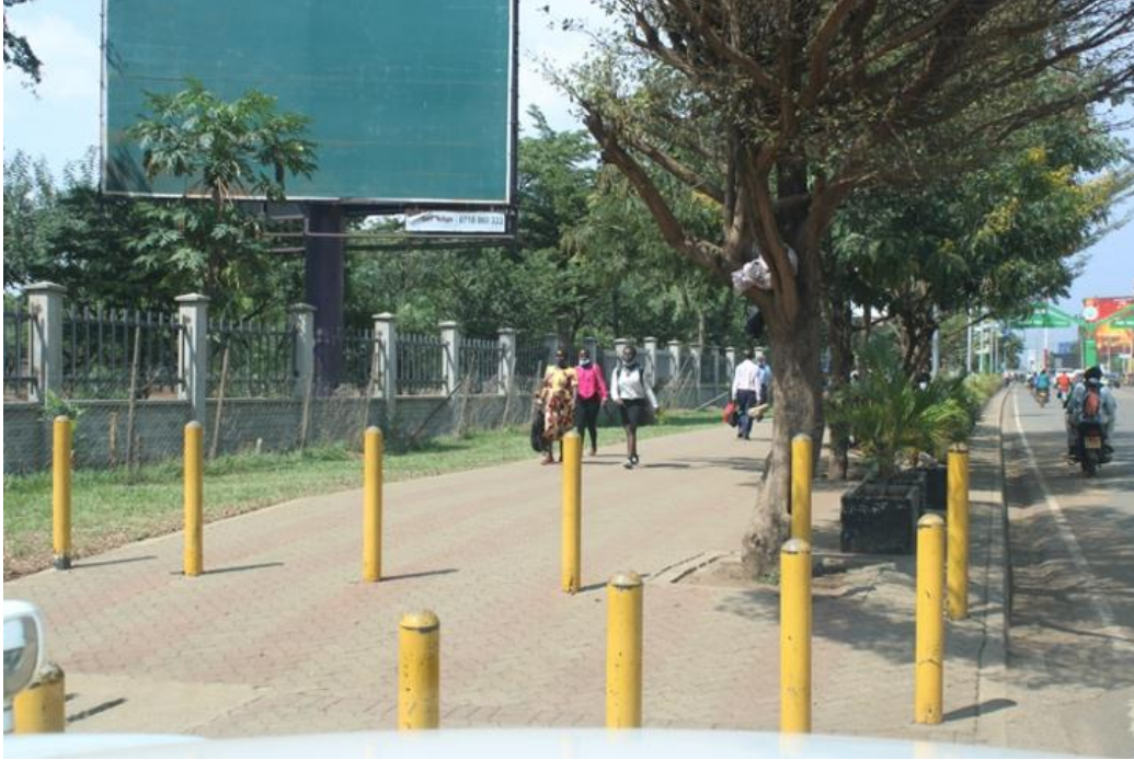
Plate 4. Retrofitted roads in the city.
