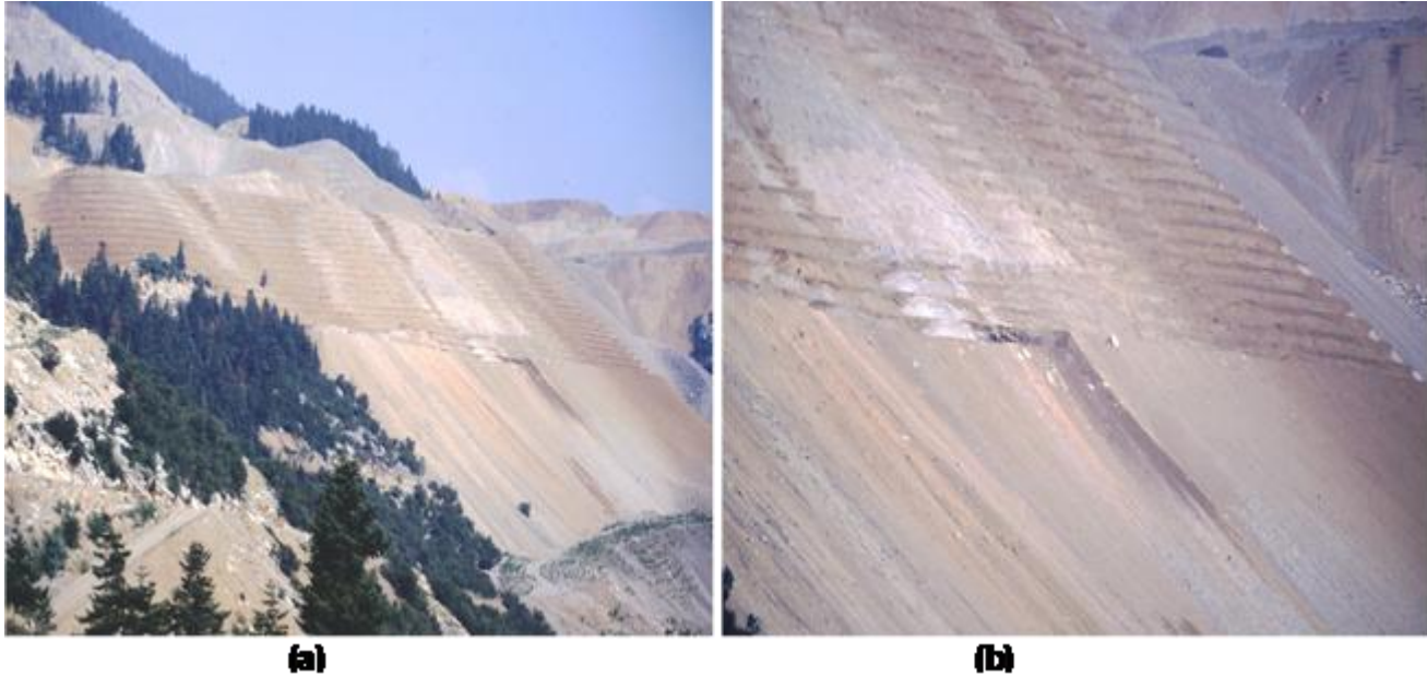
Figures 9. (a) Inert materials deposits (bauxite mining spoils) on Koukouvista 5 opencast mine, at an early stage of restoration. (b) Detail of the restoration terraces construction by earthmoving machinery-excavator (Mertzanis et al., 2004a).
