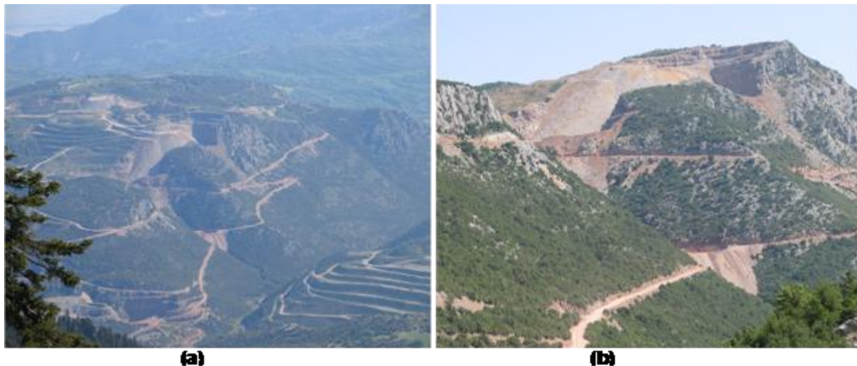
Figures 10. (a) Dense road network constructed in order to get access to the Kokinovrahos opencast mine (Mertzanis et al., 2005b). (b) Obstruction of water courses due to deposition of inert material inside the streambed, in the Kokinovrahos opencast mine area (Mertzanis et al., 2004a).
