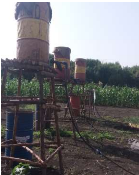
Figure 3. Field layout of family drip irrigation system.
