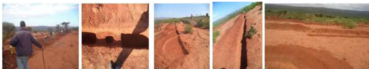
Figure 2. Constructed moisture conservation structures in the selected site.
