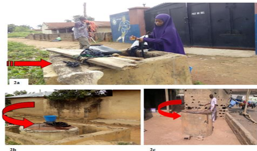
Figure 2. The diagrams of wells and pits in close proximity in the studied area.
