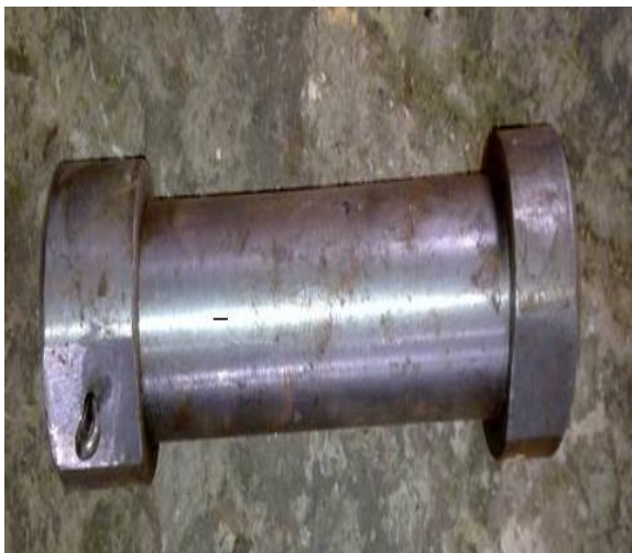
Figure 4. Longitudinal crack in cage pin with nut.
