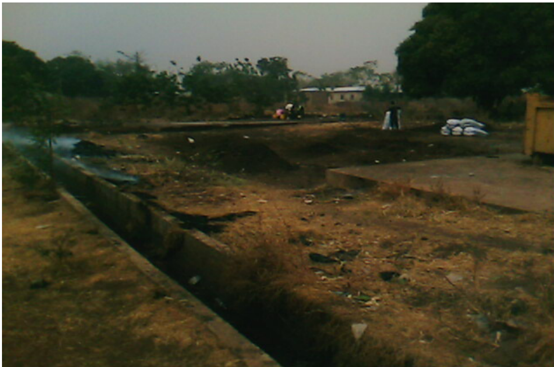
Figure 3. External drain carrying effluent towards community.
