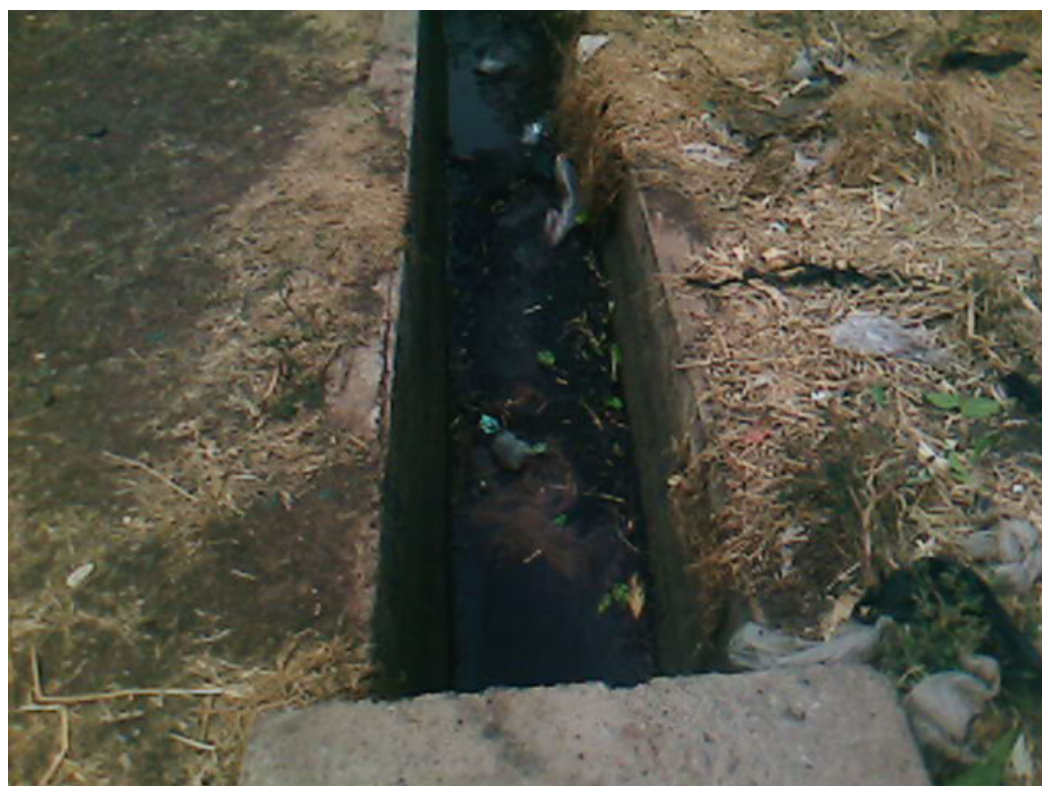
Figure 2. External drain carrying effluent from abattoir.
