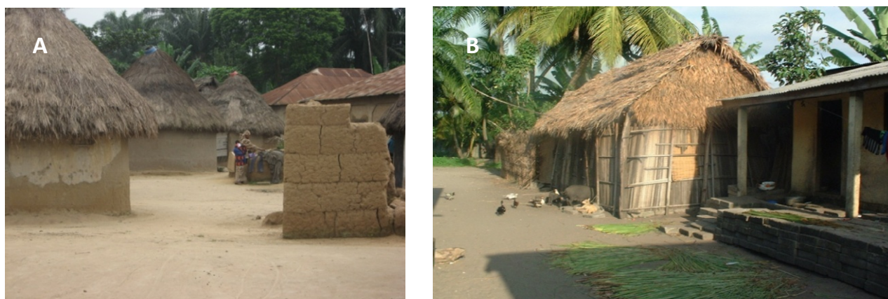
Figure 2. A) Mud habitats at Dangbo; B).Habitats of bamboo and concrete built side by side in the Aholouyeme district of Seme.
