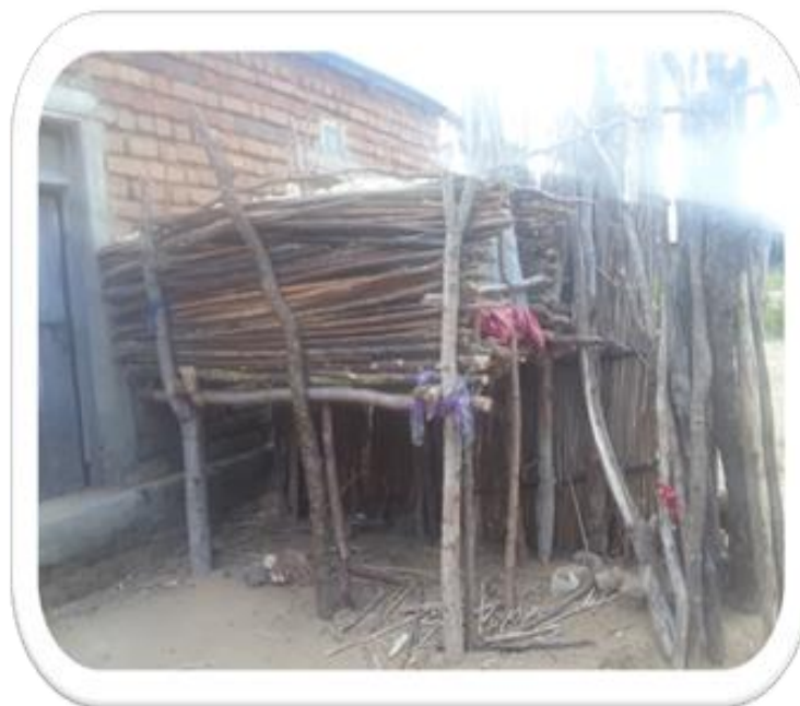
Figure 4. Homemade gallery for drying and temporary storage “Haubi” village, Kondo district Source: Author survey (2021).
