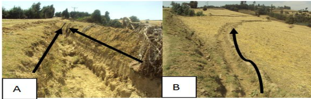
Figure 2. (A) Water way and (B) Cutoff drain.
