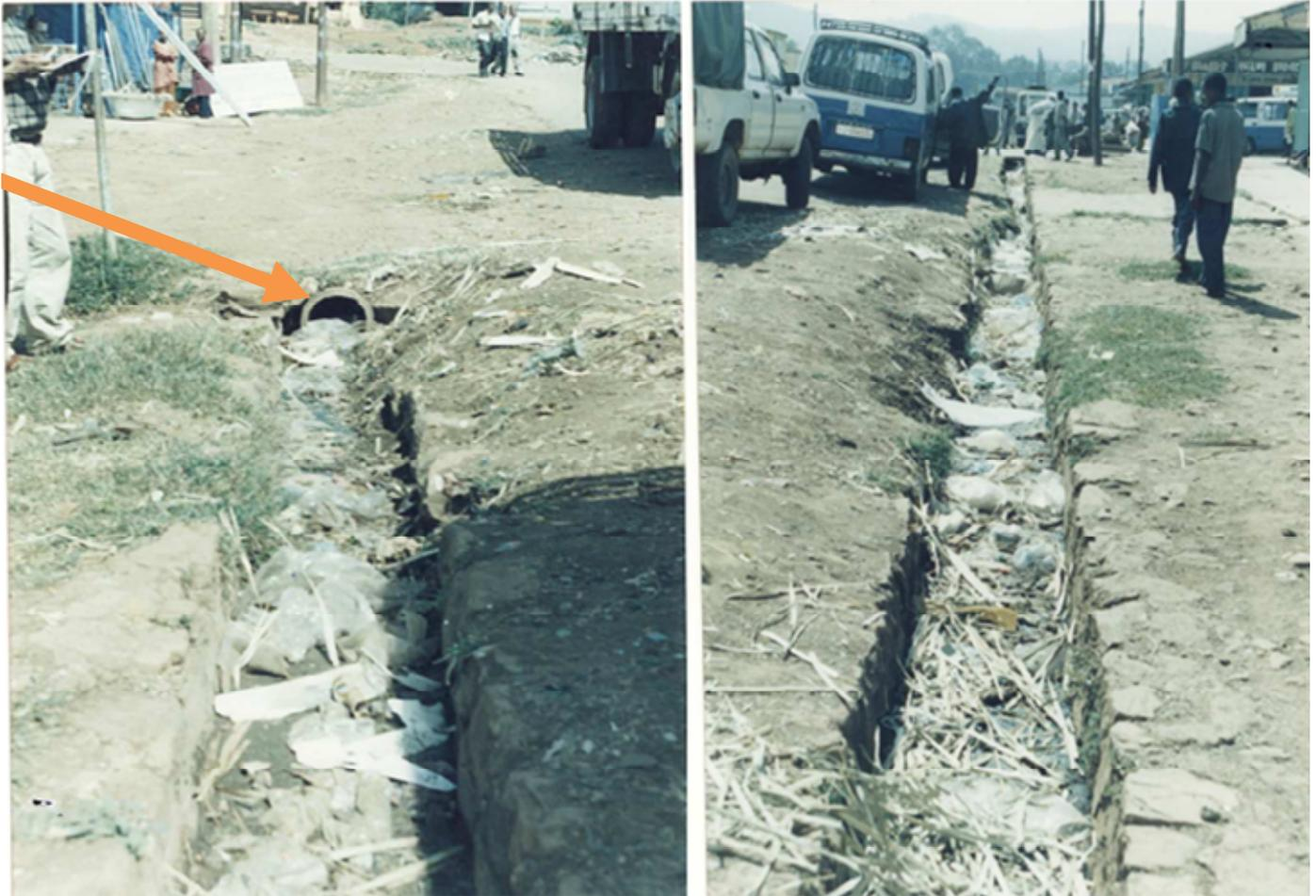
**Figure 3.** Plastic bag wastes clogging sewerage lines (or drains) (in Jimma City).
