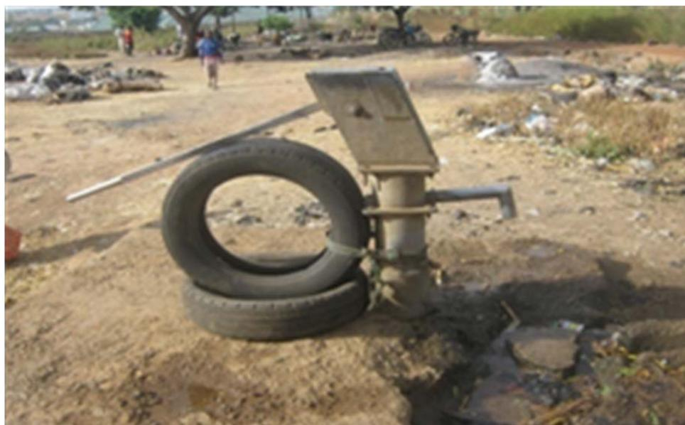
**Figure 1.** Hand pump borehole as a source of water.
