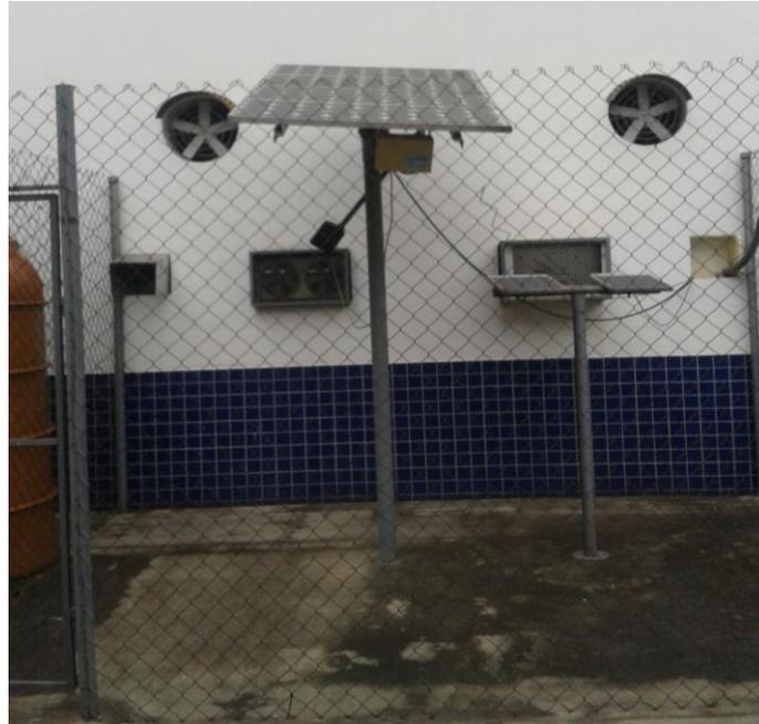
**Figure 3.** Photovoltaic panels to power an air conditioning system.
