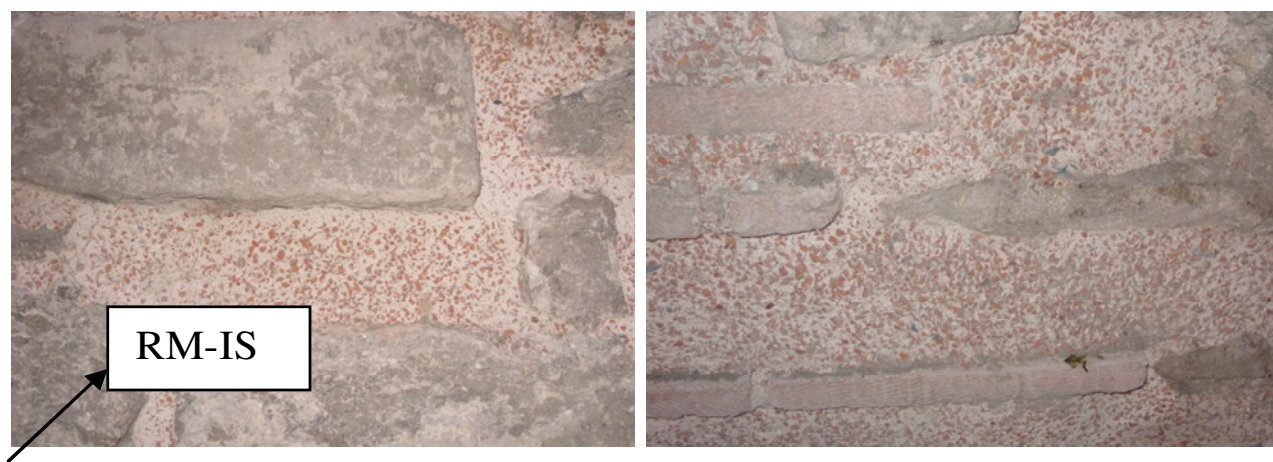
Figure 9. Location of the sample taken from the repair mortar which is previously used in the restoration of Anemas Dungeons.
