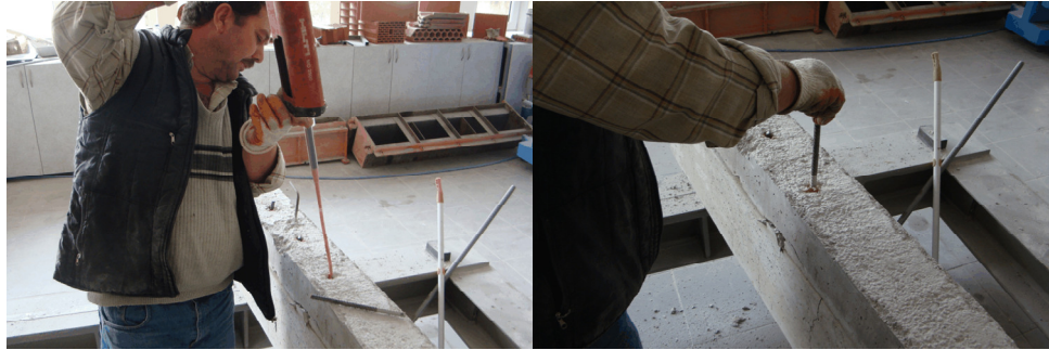
Figure 2. The implementing of Hilti and anchorage rods.
