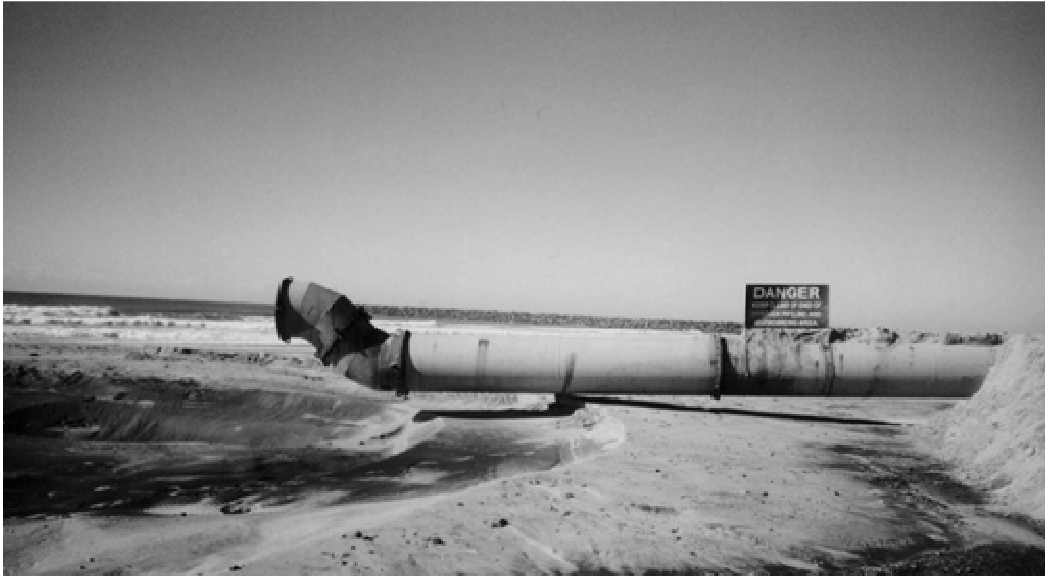
Figure 3. Outlet of the dredger pipeline that carries the polluted and sandy waters of the port entrance back onto the public beach at Alkanstrand. To compensate for the erosion due to the breakwaters trapping the coastal drift, this pipeline allows the regular fortification of the beach.
