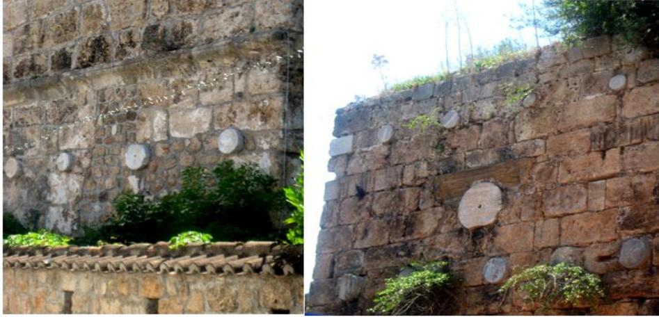
**Figure 16.** (Left) a general view of the spolia columns vertically integrated to masonry. (Right) spolia columns with changing diameters integrated to the fortifications of the citadel of Antalya (Attaleia), southwestern Turkey (Construction date: Anatolian-Seljuk period, early 13<sup>th</sup> century / photograph by Kavas (2012).
