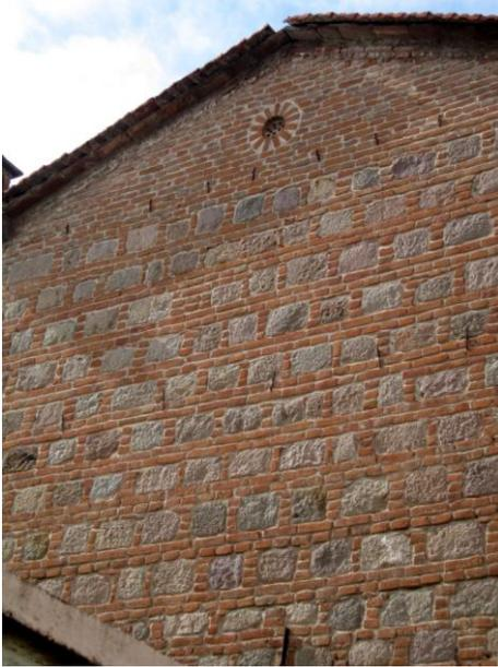
**Figure 22.** Combination of brick and stone (alternative wall) in a dwelling wall in Bergama (Ancient Pergamon), western Turkey, (Construction date: early 20<sup>th</sup> century, photograph by Kavas (2012).
