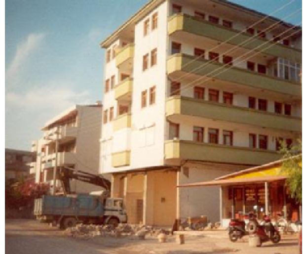
Figure 5. Structurally damaged five-story reinforced concrete building located on liquefiable soil.
