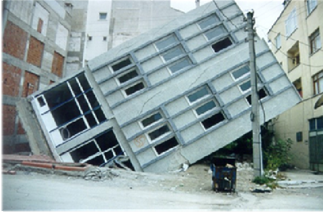
Figure 3. Totally damaged structure built on liquefiable soil.
