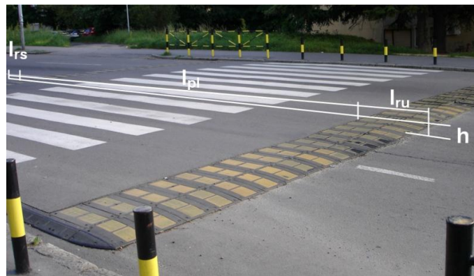
Figure 5. Speed control hump - flat platform.
