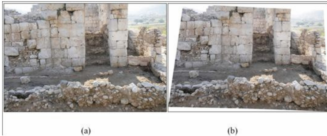
Figure 7. (a) Raw images from Patara Hurmalik Bath, control points on the buildings and rectified image. (b) Images obtained by laser scanning.
