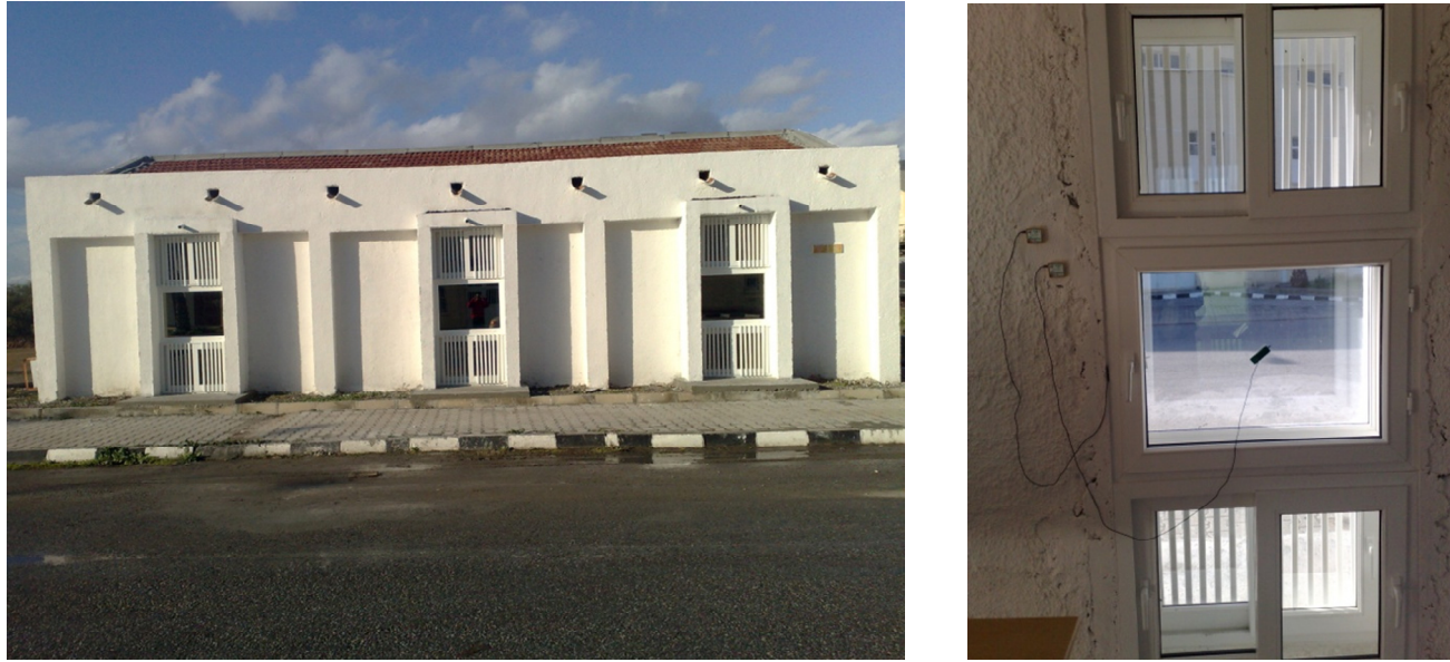
Figure 2. Pictures from outside and inside of the south facade of the test house.
