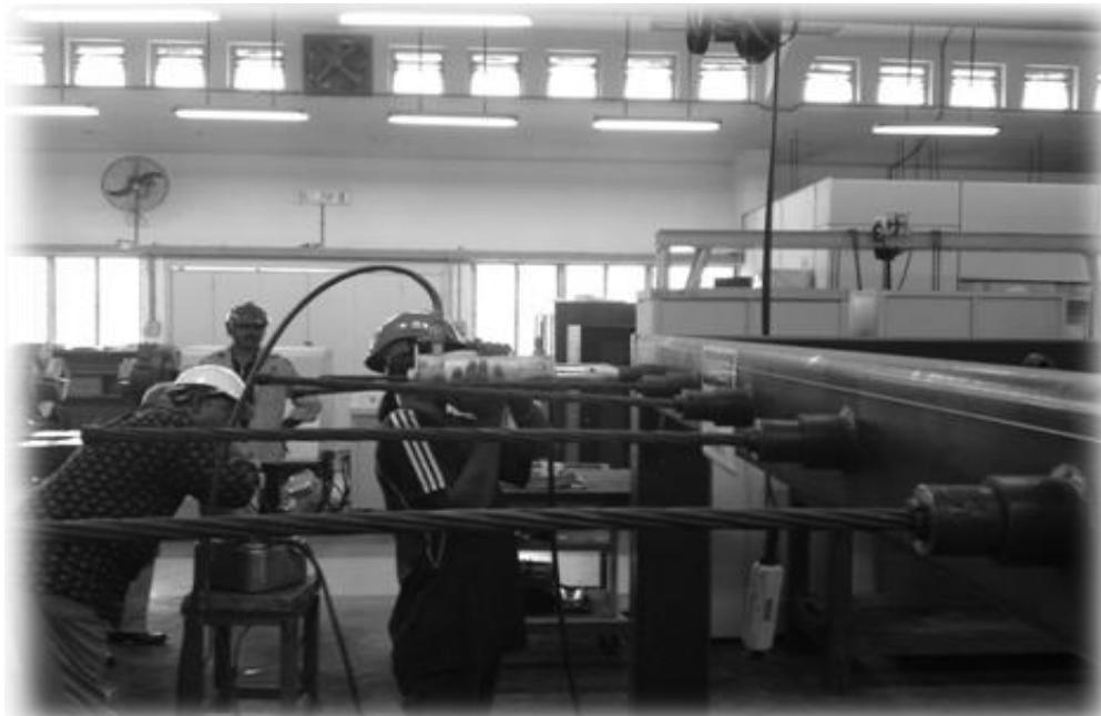
Figure 3. Construction of frame steel.
