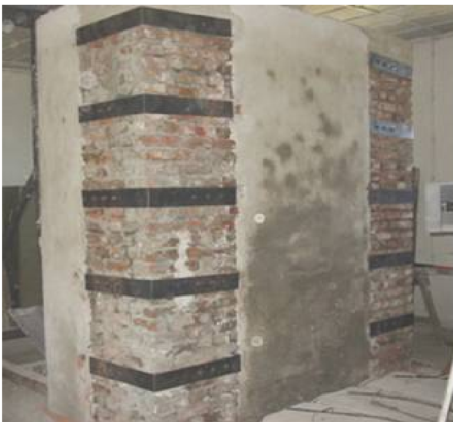
Figure 8. The application of L-shaped reinforcing plates from outside of the wall.
