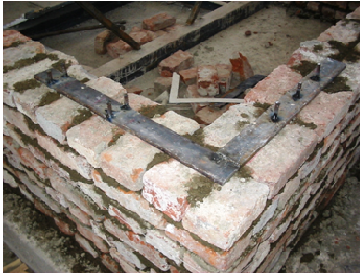
Figure 5. The applications of L-shaped corners bars.
