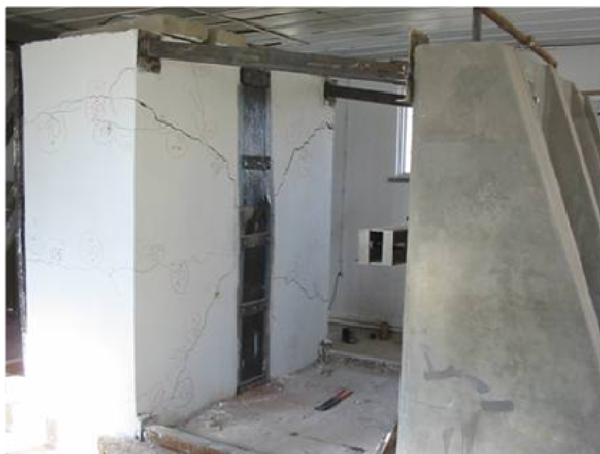
Figure 11. The masonry wall strengthened by FRP-sheet at centre: Wall D.
