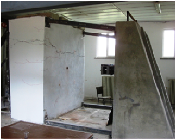
Figure 7. The cracking pattern of Wall B corresponding to ultimate stage.
