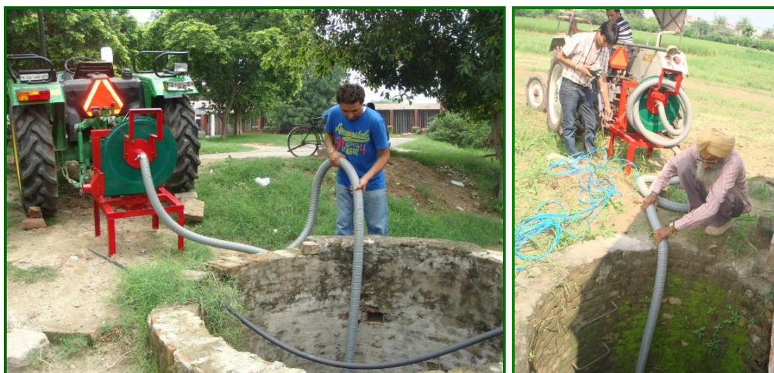
**Figure 5.** Measurement of CO<sub>2</sub> concentration during removal of gases from tubewell pit
