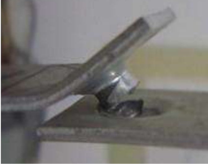
Figure 2. Typical failure modes of SPR joint: rivet tail pull-out.
