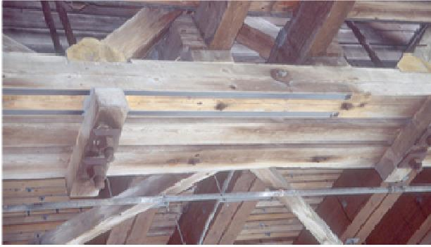
**Figure 1.** Restrengthening of bottom chords of the timber bridge (Steiger, 1999).
