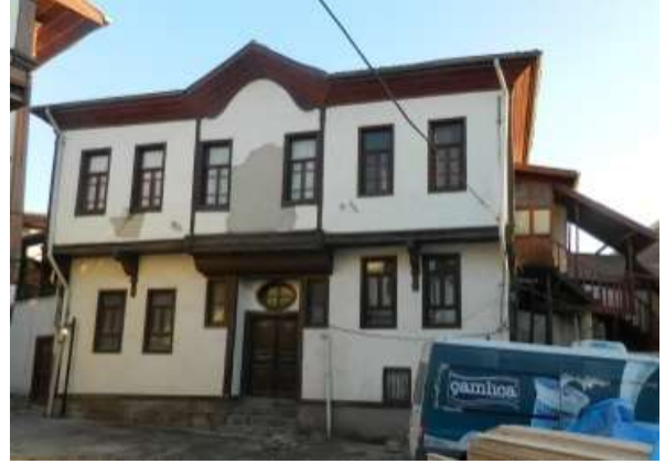
Picture 28. The cement stucco (Source: Writer, 2014).
