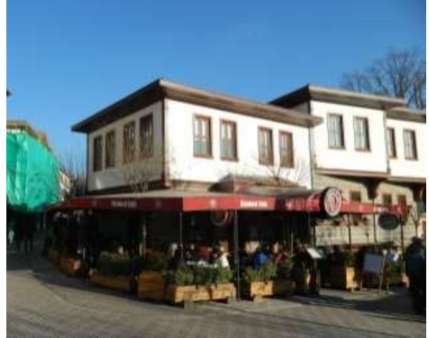
Picture 32. Current status of the house (Source: Writer, 2014).
